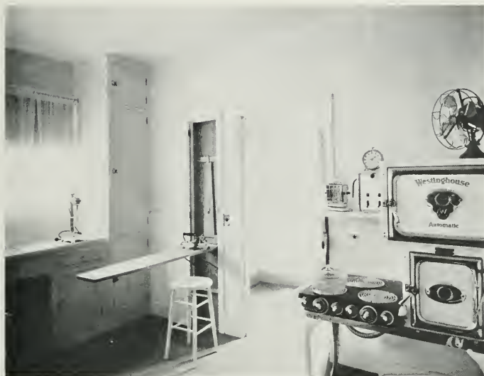
KITCHEN, COMPLETE ELECTRICAL HOME, SAN FRANCISCO
