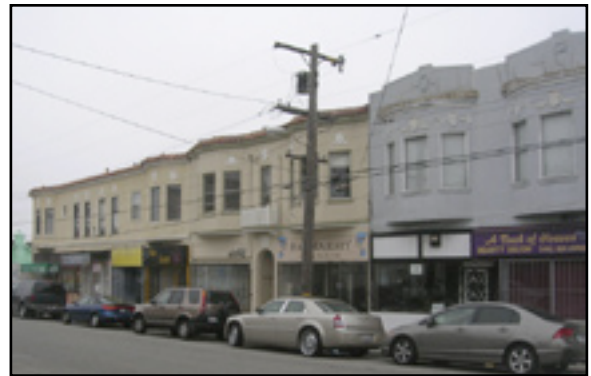
Ingleside, commercial: 800 block of Holloway, built 1926
