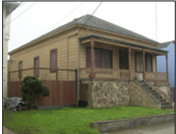
Ocean View residential: 227 Sadowa Street, built 1910
