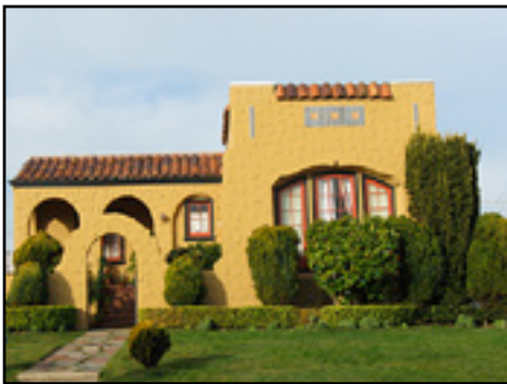
Ingleside Terraces single-family: 85 Borica Street.
