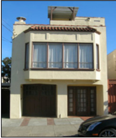
Ingleside residential: 306 Ashton Avenue, a 1923 building in the style of a Sunset District row house with equal visual emphasis given to the garage and pedestrian openings.
