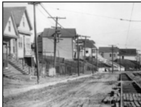
Homes on San Jose Avenue near Lakeview Avenue, 1922. (Courtesy of Western Railway Museum.)
