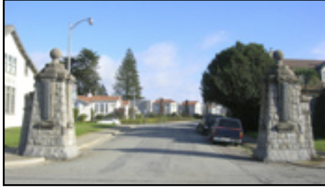
Ingleside Terraces monuments: pillars at Estero Avenue near Junipero Serra Boulevard.
