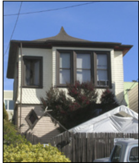
Ingleside residential: 146 Beverly Street, built in 1914. Surrounded by houses built in the 1940s
