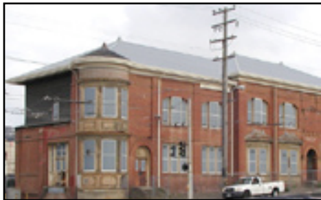
Geneva Office Building, 2008.
