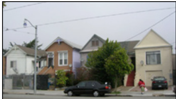
Ocean View residential: four Victorians on Broad Street, connected to Spring Valley water service during the 1890s.
