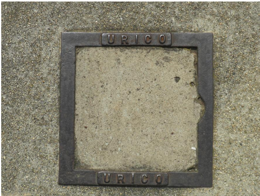
A cement filled drain cover: one of the few remaining records of the Urban Realty Improvement Company (URICO) at the site. Four can be found near where the reflecting pool used to exist and one other nearest the southern entrance of Entrada Court. (Derek A. Cinpak, 5 Apr 2011)
